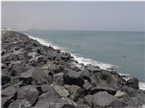
Photo 3. The fixed nets along the dike.
