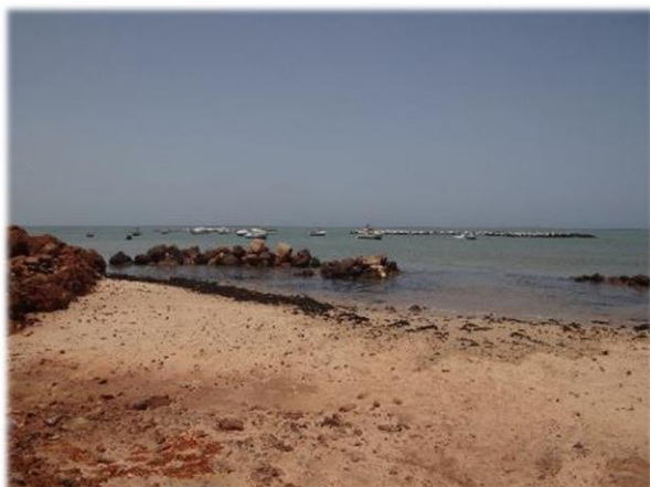
Photo 3. The seawalls financed by the AF project in Saly.
