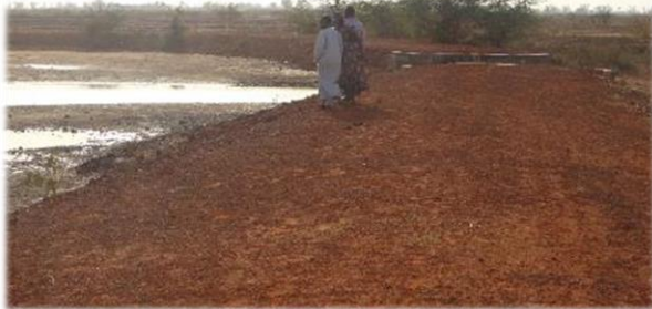
Photo 11. The water discharge basin on the anti-salt dike whereby the right and left banks meet, seawater is retained between the two openings and fresh water is retained upstream during precipitation.
