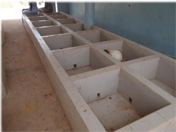
Photo 8. Under-utilised washing basins fitted with a water drainage system financed by the AF project.
