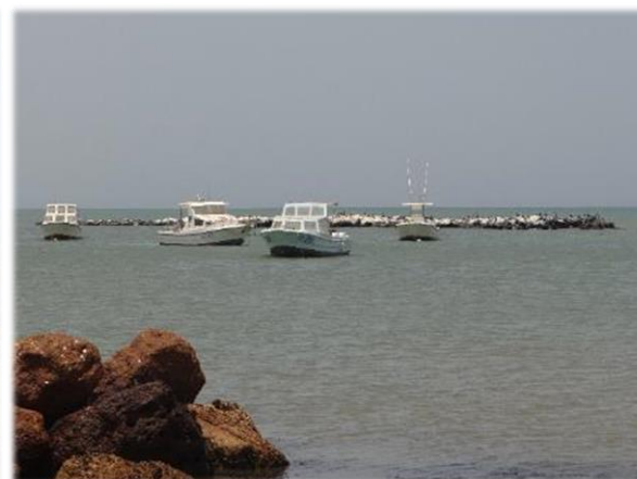
Photo 4. A seawall constructed in Saly.
