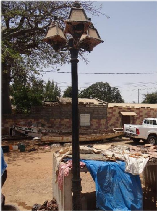
Photo 12. Solar lighting system financed by the AF which is no longer functional.
